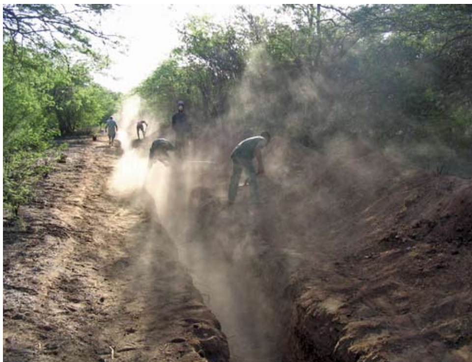
DIGGING THE TRENCHES FOR THE INFRASOUND ELEMENTS OF IS11, CAPE VERDE, DECEMBER 2006
