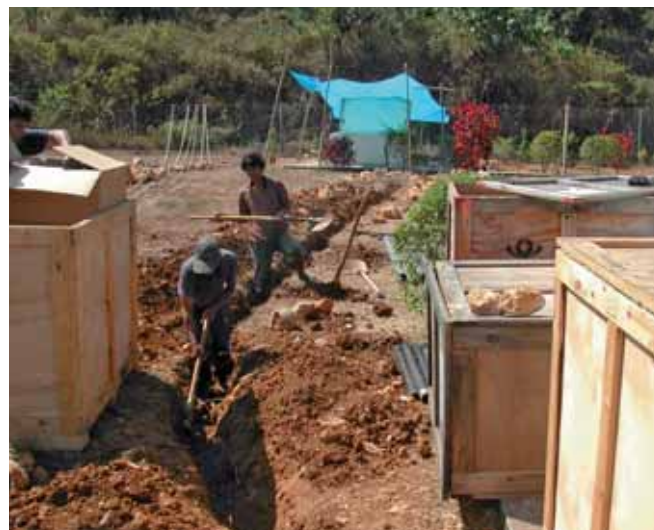
DIGGING A TRENCH FROM THE SENSORS TO THE CENTRAL RECORDING FACILITY, AUXILIARY SEISMIC STATION AS44, KAPPANG, INDONESIA
